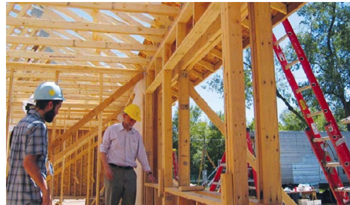
The NREL/Habitat Zero-Energy Home utilizes double-stud walls that leave more room for insulation than regular single-stud walls.
