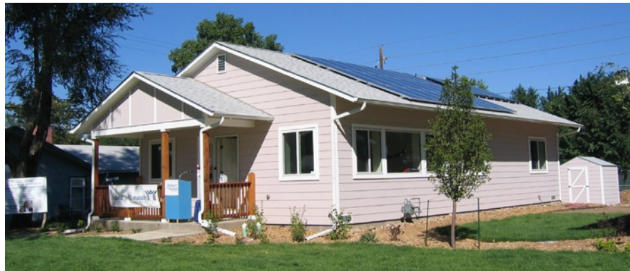
The 1,200 sq ft home uses passive and active solar features to help reach the zero energy goal.
